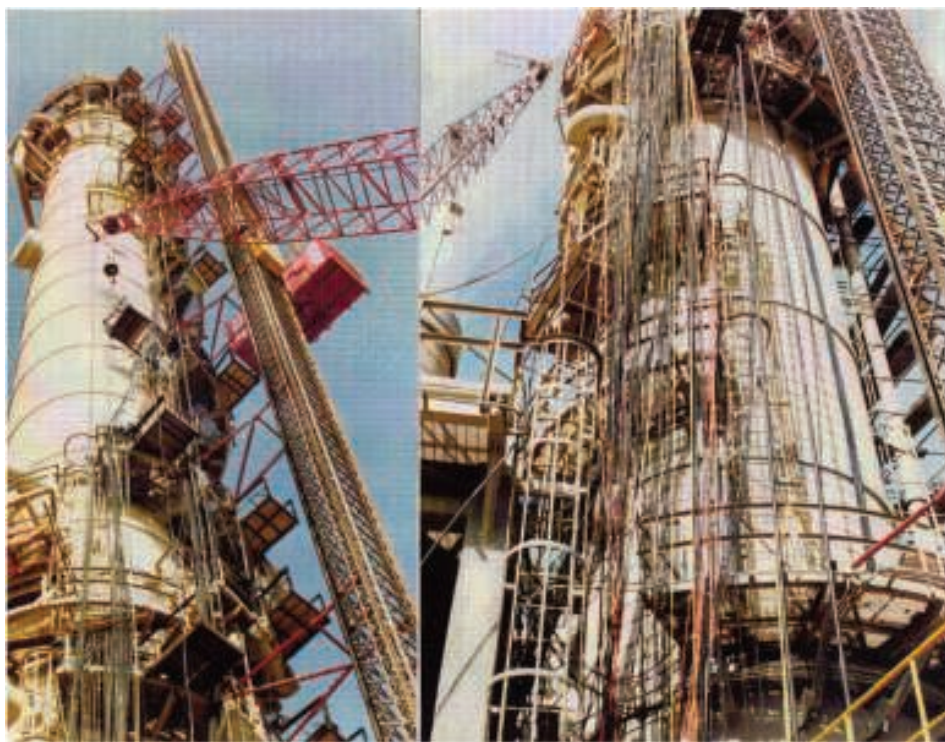
FIGURE 1. Revamping a column is a major undertaking
